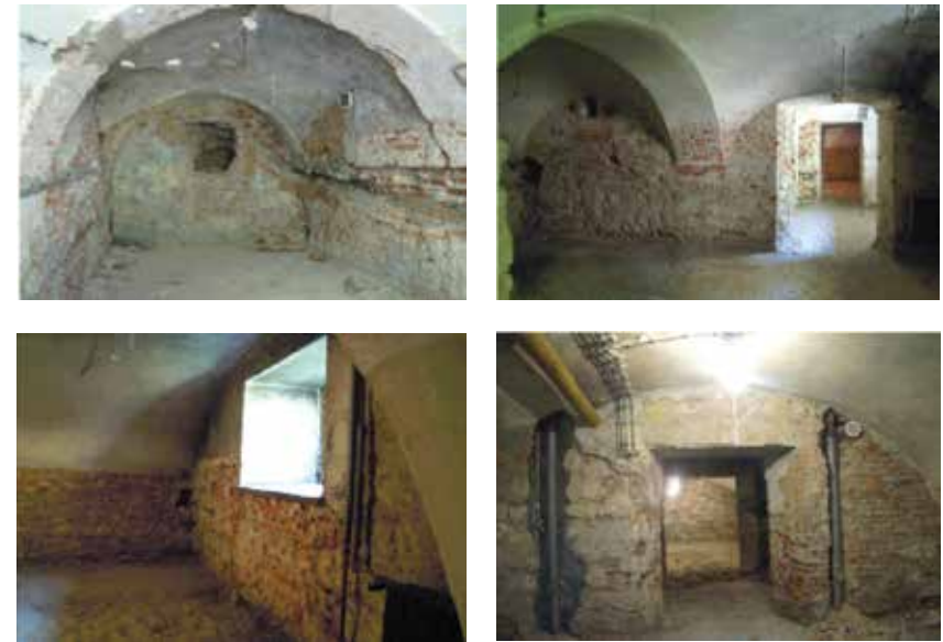
Basement of the building located at 7 Kopernika St, Krakow before its full renovation in 2011
